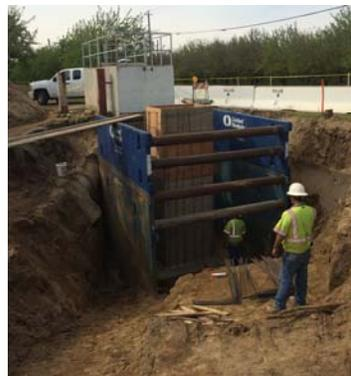
Photo Left: District crews building float box on the H line to control water levels passing through.
